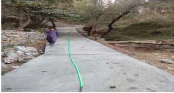
Batangi Road after Completion
